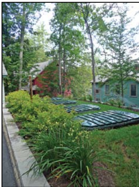
Advanced systems such as this Puraflo system that uses peat moss can help get around physical constraints such as small lot size or bedrock.
