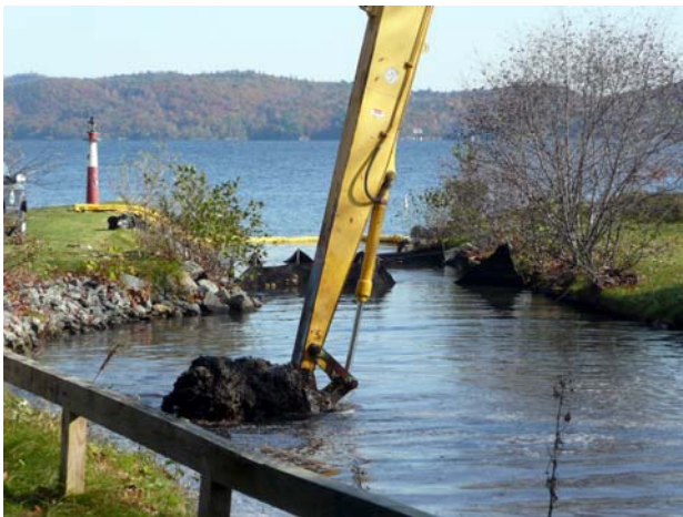
Photo caption: A long-reach excavator removes sediment from a retention basin at the mouth of Jenkins Brook.
