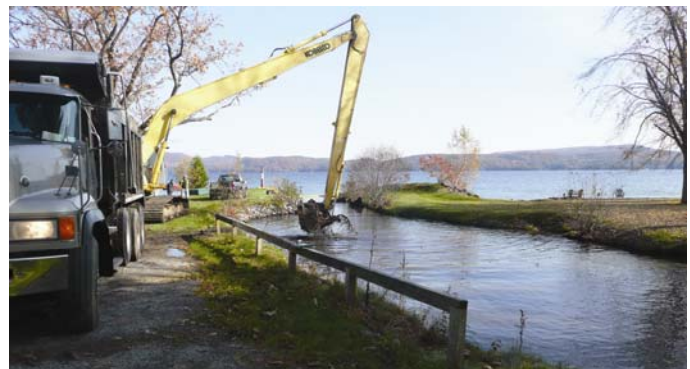
Photo caption: A long-reach excavator removes sediment from a retention basin at the mouth of Jenkins Brook.
