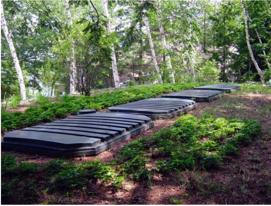
Picture one caption: Alternative peat bio-filter septic systems, like the one pictured here, are just one of several green landscaping technologies that will be showcased at the LGA's upcoming open house. These systems are ideal for difficult sites – small lot-size, high bedrock – and provide superior wastewater treatment.
