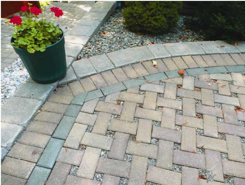
Picture two caption: Replacing impermeable asphalt with permeable pavers, like those pictured above, can significantly reduce stormwater runoff problems on steep sites, while enhancing the aesthetics of any landscaping project.
